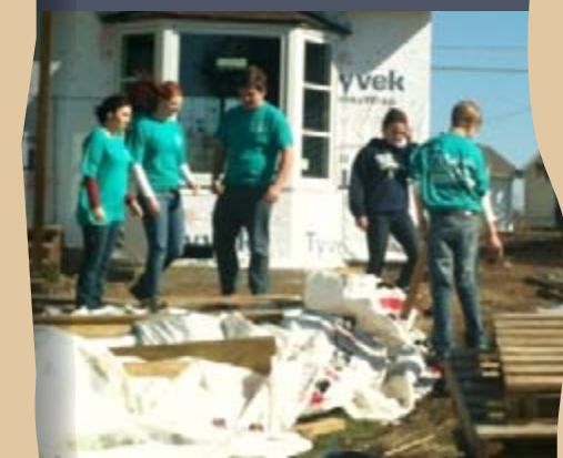
Catholic Charities workers and volunteers help to rebuild a house in Joplin.
