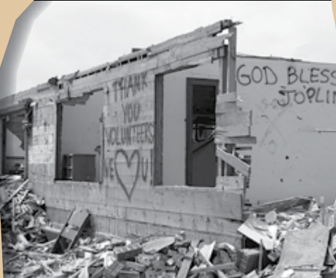
What's left of a home in Joplin, Missouri after a deadly tornado.
