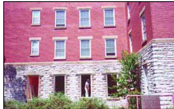
La Salle Retreat Center New Windows — West Wing
