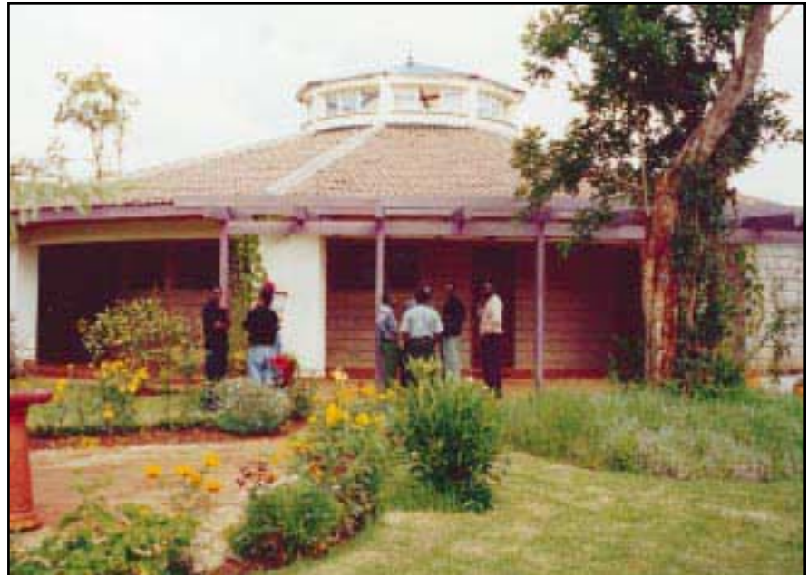
Scholasticate chapel building in Nairobi, Kenya, Africa
