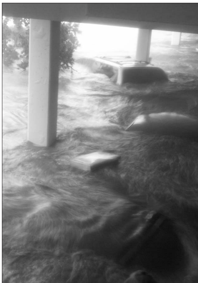
Storm surge at St. Stanislaus College Preparatory High School, Bay Saint Louis, MS.
